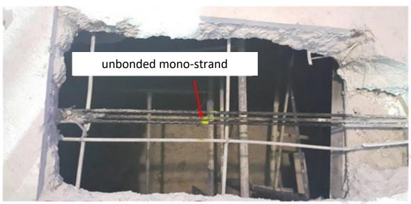
4. Cut strand after install temporary locking equipment and then release force in strand and move temporary locking out.
